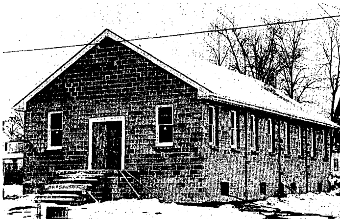
Hightstown Assembly under construction; P. Gibilisco, Pastor
